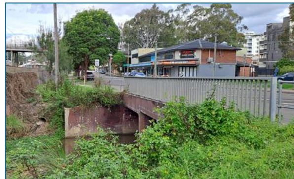
Looking south across Girraween Ck from the existing railway underpass to the 'shared path' along Portico Pde. A bridge in parallel to the road bridge would improve connectivity for pedestrians and riders.
