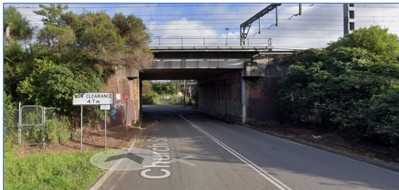
Google Streetview image of the Church St railway underpass.
