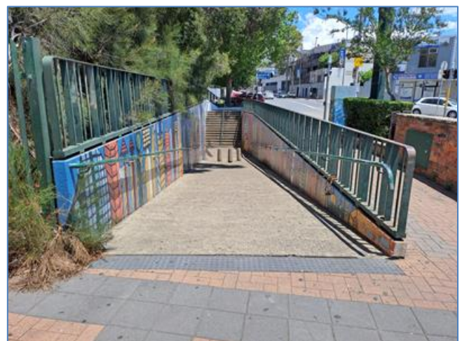
Western-side ramp to underpass at Merrylands Station where riders are instructed to dismount and walk. The ramp has offset bollards at the bottom which may be tricky to negotiate for some potential users.
