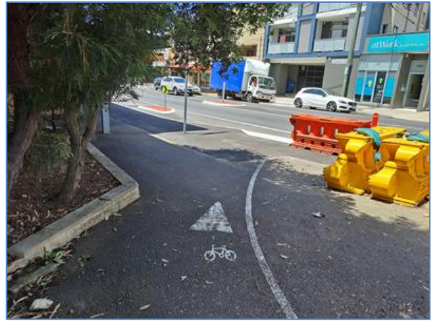
Cyclists appear to be directed onto the road just before a barrier in the shoulder lane.
