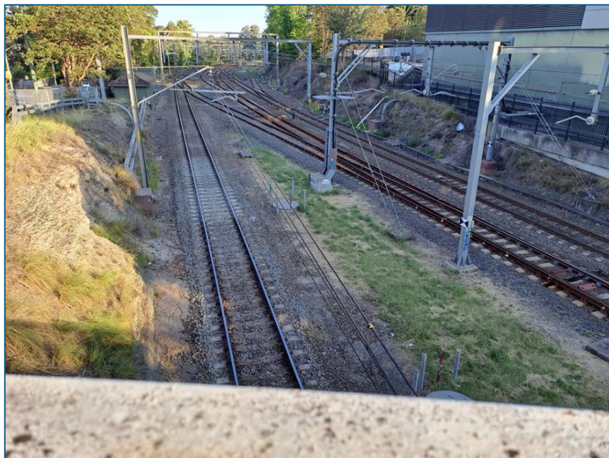
Looking over railing on existing bridge to grassed area in between lines where platforms 1 & 2 could potentially be extended, with lift access up to new bridge.
