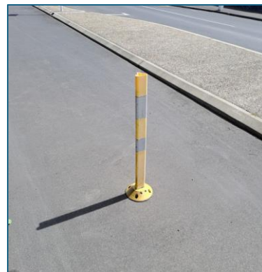
A Flexible bollard on a separated cycleway in Dunedin, NZ.
