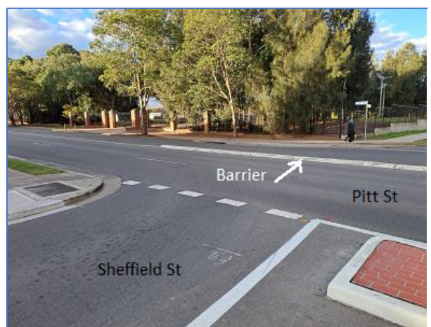
Low level barrier on Pitt St for riders crossing or needing to cross when turning.
