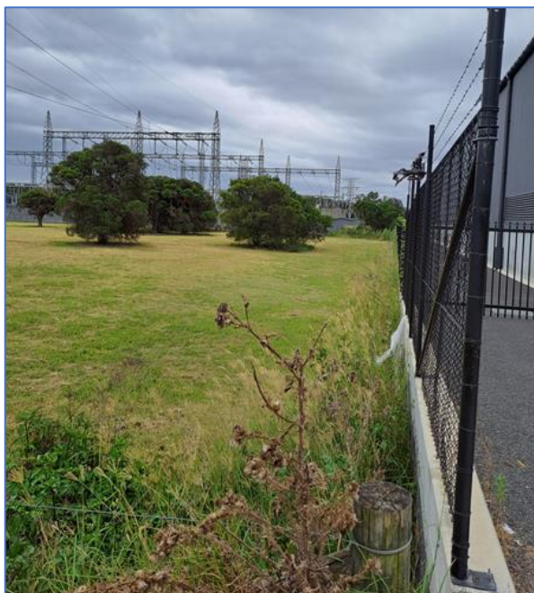
Looking north from Yarrawa St into the proposed corridor on the substation land which borders the new complex at 5 Yarrawa St.
