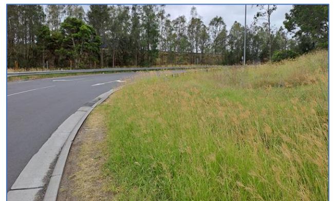
Crossing M7 northbound exit ramp (Points E to F on above image).
